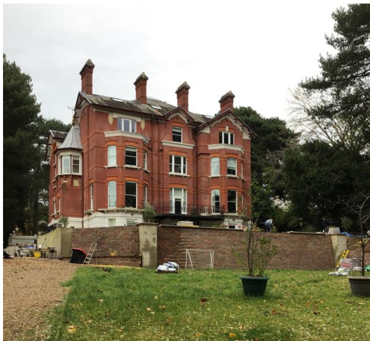
Figure 2: Rear of the site looking back onto No.54:
